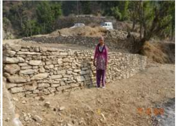
Retaining walls/check dam
